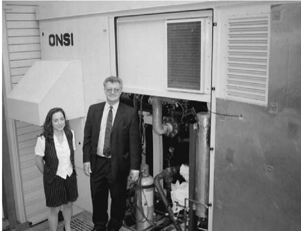
Fig. 1. Mr. Allan Jones, the Energy Services Manager of the Woking Borough Council, spearheaded the implementation of Britain's first commercial combined heat and power fuel cell system. The 250 kW ONSI unit, produced by International Fuel Cells Inc., began in 2002 to provide heating, cooling, and electricity to Woking Park's swimming pool and leisure complex. Shown with Colella.
